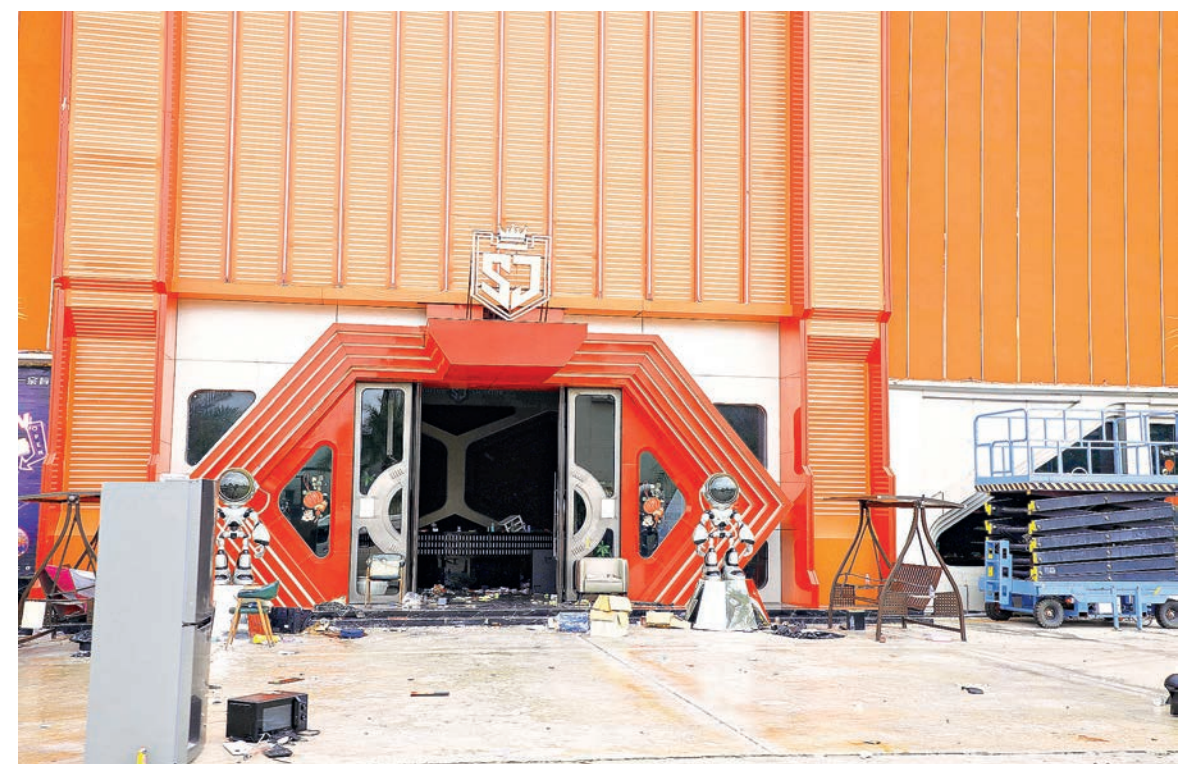
This photo reveals the ongoing demolition measures.
