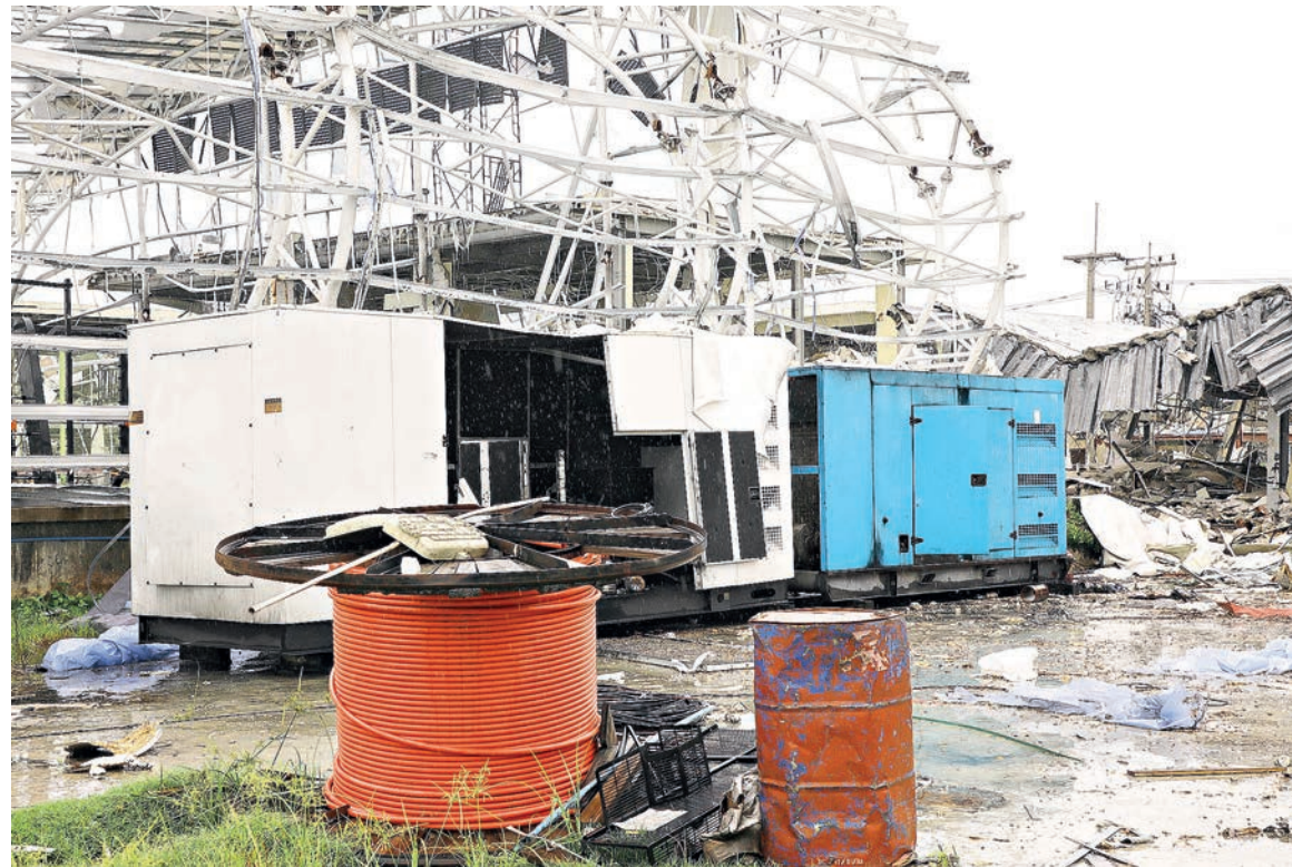
This image shows the demolition process.
