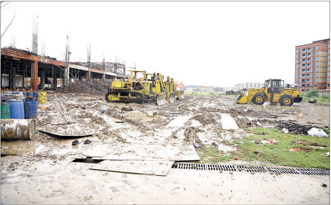
The ongoing demolition measures in the KK Park area.
