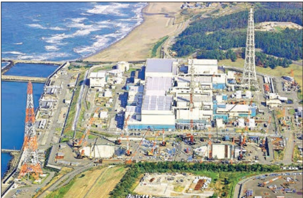
Local governor's approval is viewed as essential for restarting the No 6 reactor, with support from the heads of Kashiwazaki and Kariwa municipalities hosting the facility. PHOTO: KYODO
