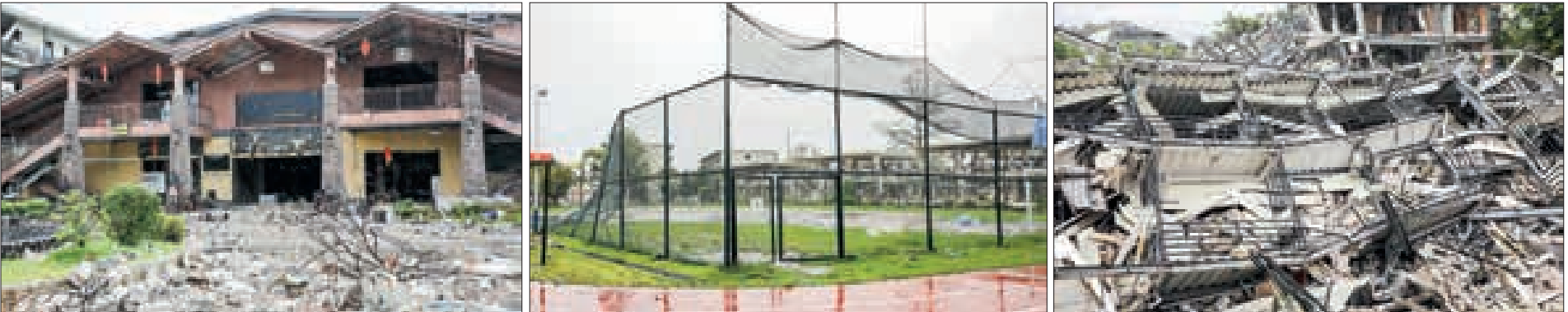
Photos show buildings and facilities in the KK Park area being demolished as part of a major crackdown on online scams and illegal gambling. PHOTO: MIN MIN
