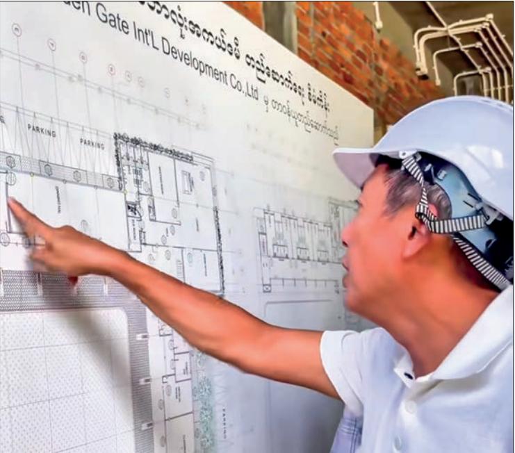
MFF President U Zaw Zaw makes a visit to the women's football academy under construction.
