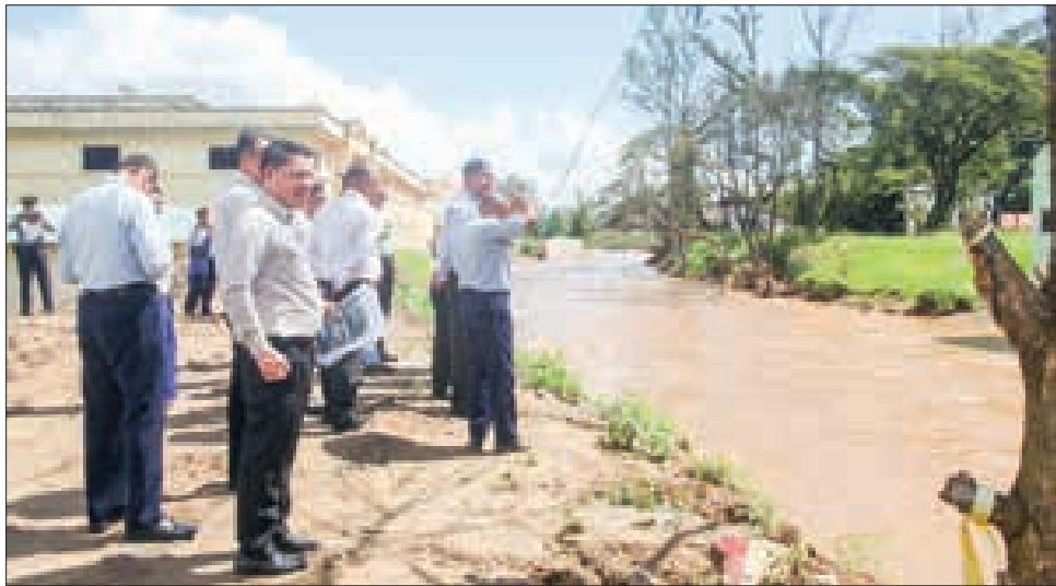
Deputy Ministers U Aung Kyaw Tun and U Myo Myint inspect the construction site of concrete retaining walls in Tachilek on 17 October 2025.
