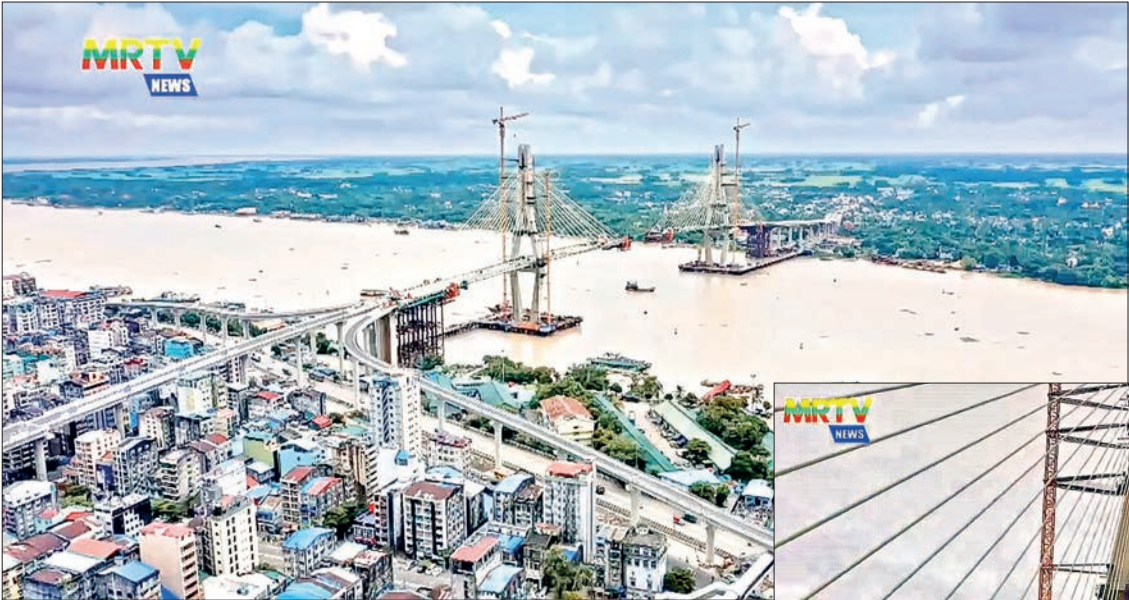
The Myanmar-Korea Friendship Bridge and the steel suspension cables.
