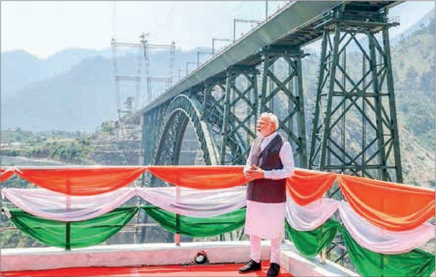
This event marks a significant milestone in improving railway connectivity in Jammu and Kashmir. PHOTO: INDIAN PRESS INFORMATION BUREAU (PIB)/AFP
