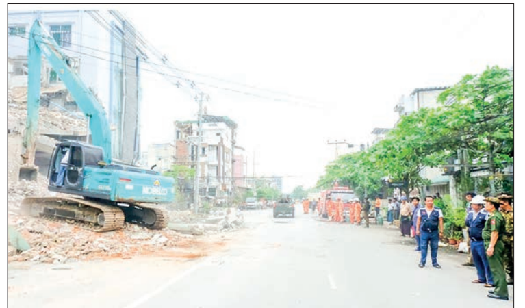
Lt-Gen Soe Tint Naing observes removing debris efforts by using heavy machines at Idea Moblie building in Chanayethazan Township, Mandalay yesterday.
