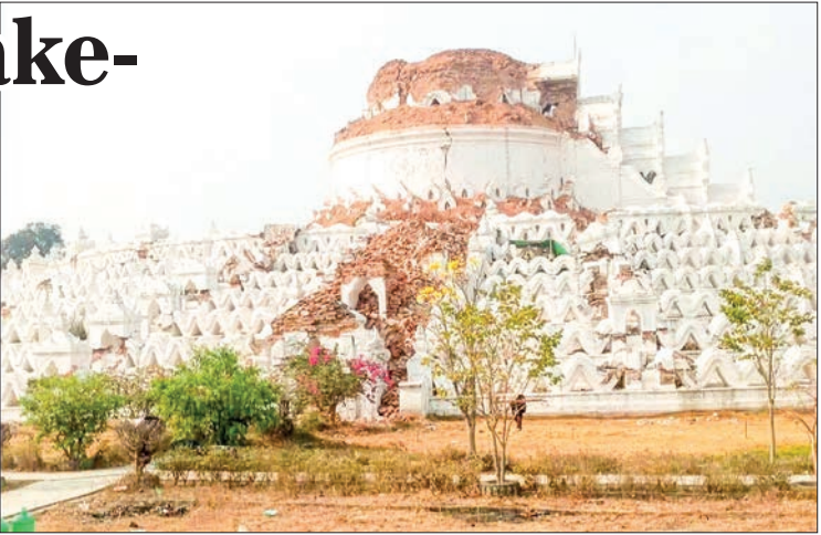
This photo reveals some of the historic structures damaged by the Mandalay earthquake.
