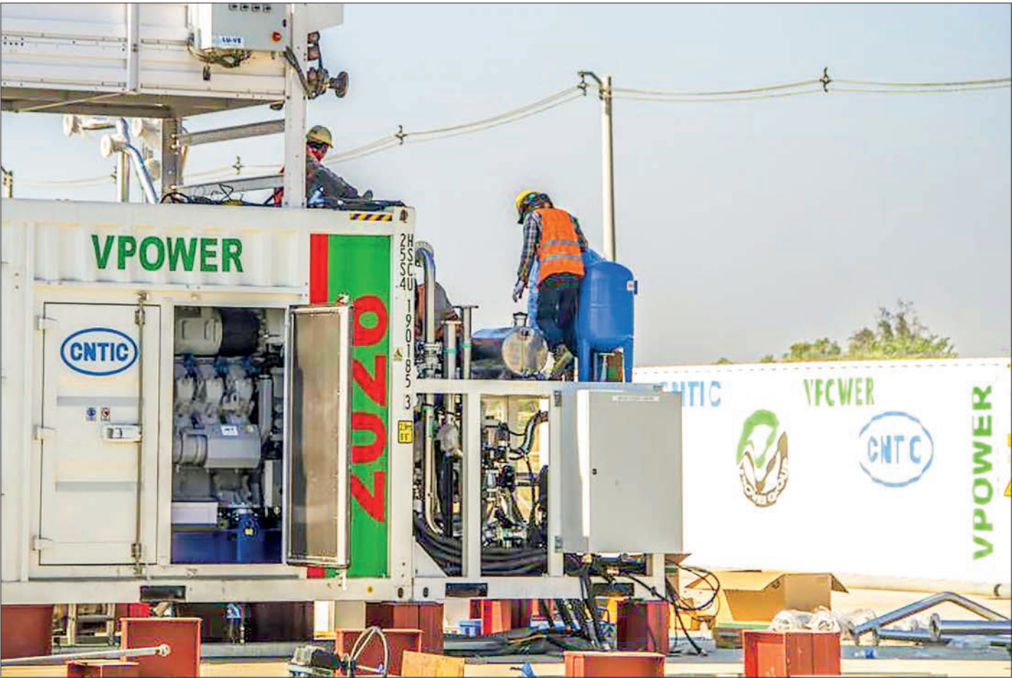
Dedicated workers labour tirelessly to restore LNG power plant operations.
