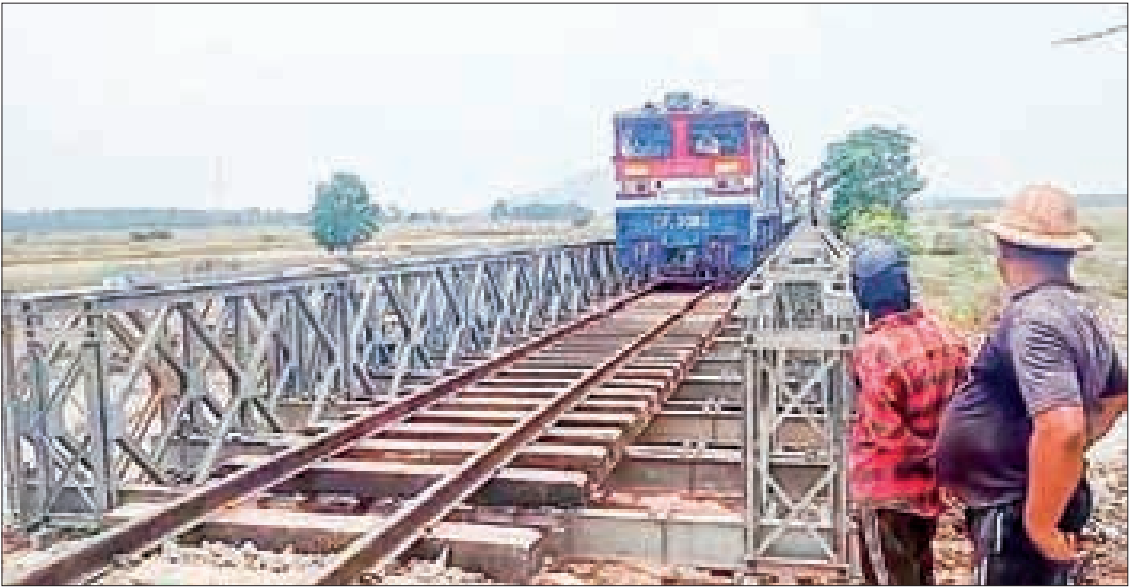
The Yangon-Mawlamyine train crosses the Bridge No 65 on the Bago-Mawlamyine railway after repairs.
