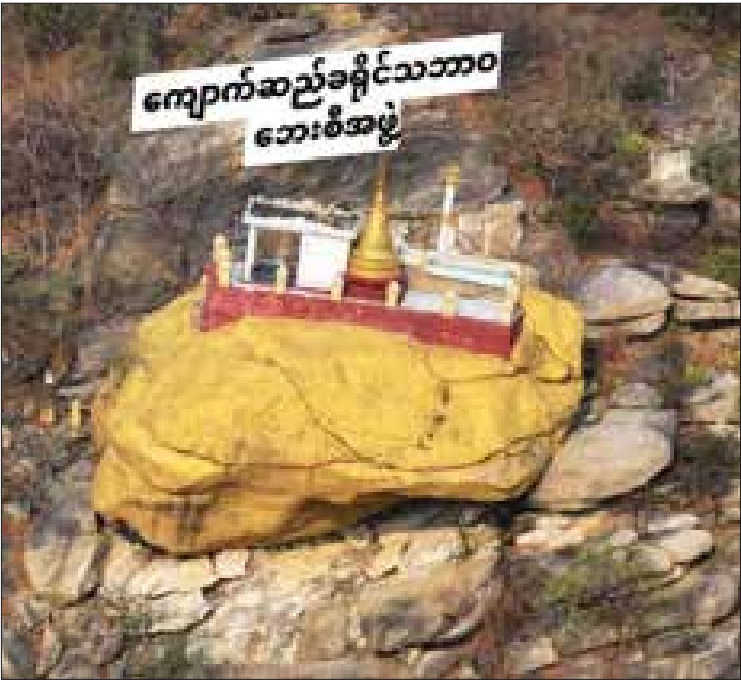
The current condition of the historic Kyaukthitta Pagoda in Kyaukse, damaged by the Mandalay earthquake. PHOTO - KYAUKSE DISTRICT DISASTER MANAGEMENT TEAM
