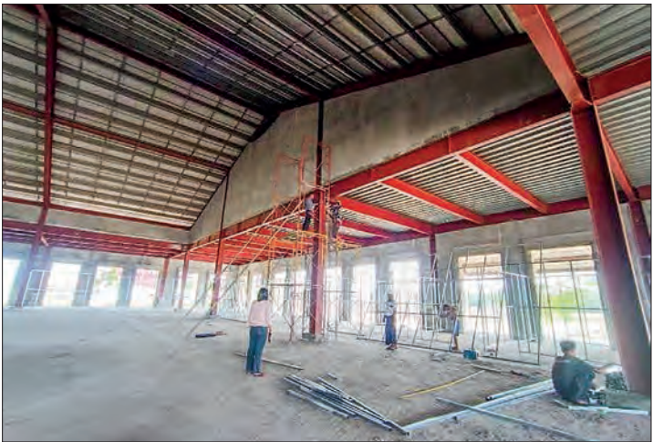
The Centre is under construction.
