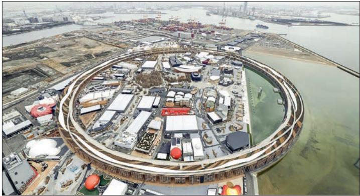
Photo taken on 12 March shows the venue of the World Exposition in Osaka under construction. PHOTO: KYODO
