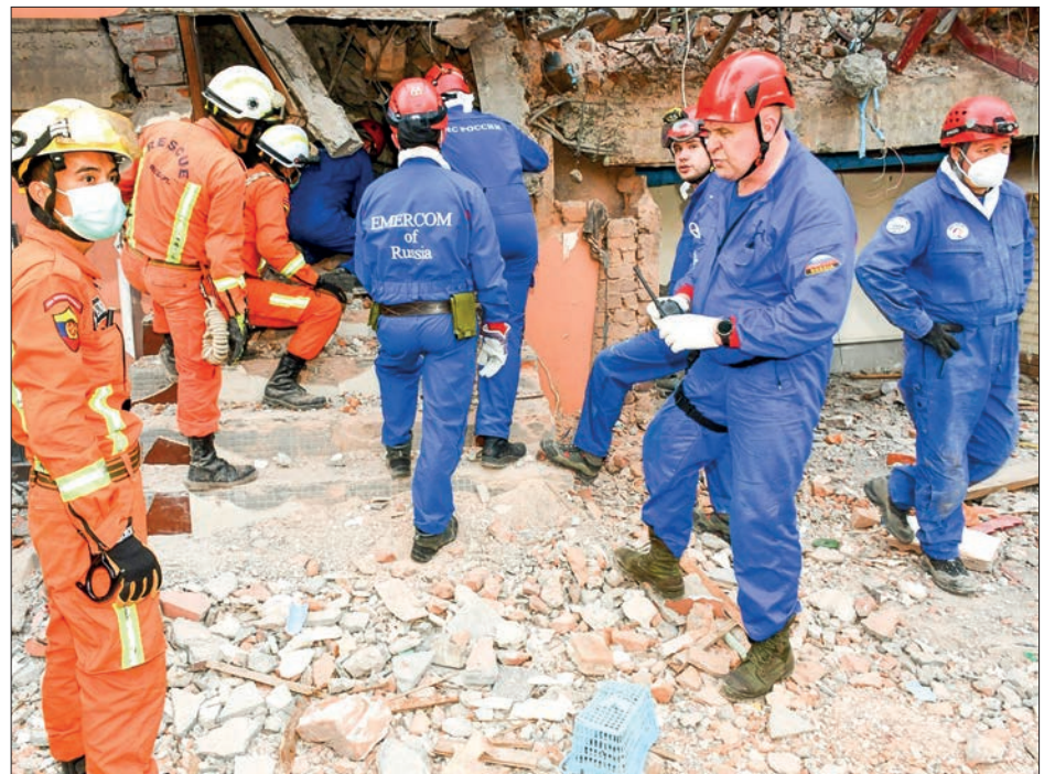
Members of Chinese and Russian rescue teams are working at the site of the collapsed Great Wall Hotel in Mandalay on 30 March 2025.
