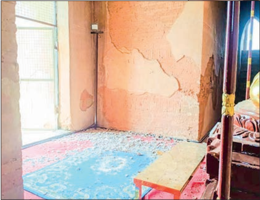
Photo shows falling some plaster of the wall of Htilominlo Pagoda. PHOTOS: ZWE MARN
