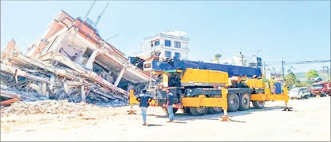
A crane from Ayeyawady Foundation prepares to remove debris in a recent earthquake struck area. PHOTO: AYEYAWADY FOUNDATION
