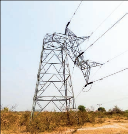
Transmission towers and facilities being damaged in the wake of powerful earthquake.
