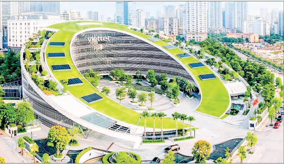
Vietnam has so far had a cumulative total of 559 green-certified buildings. PHOTO: ILLUSTRATIVE PHOTO COURTESY OF THE COMPANY VIETTEL
