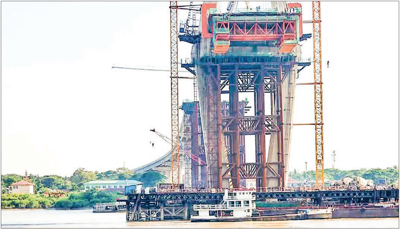
The photo shows the Yangon-Dala Bridge construction site.
