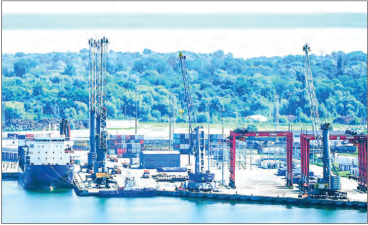
The new Ursa Major cargo ship is loaded at the Baltiysk Sea Port, where the Baltiysk - Ust-Luga ferry service is carried out, in Kaliningrad region, Russia. PHOTO: SPUTNIK/FILE
