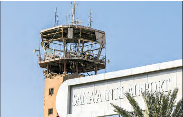
The damaged control tower at the international airport in Yemen's rebel-held capital Sanaa, after Israeli air strikes. PHOTO: MOHAMMED HUWAIS / AFP
