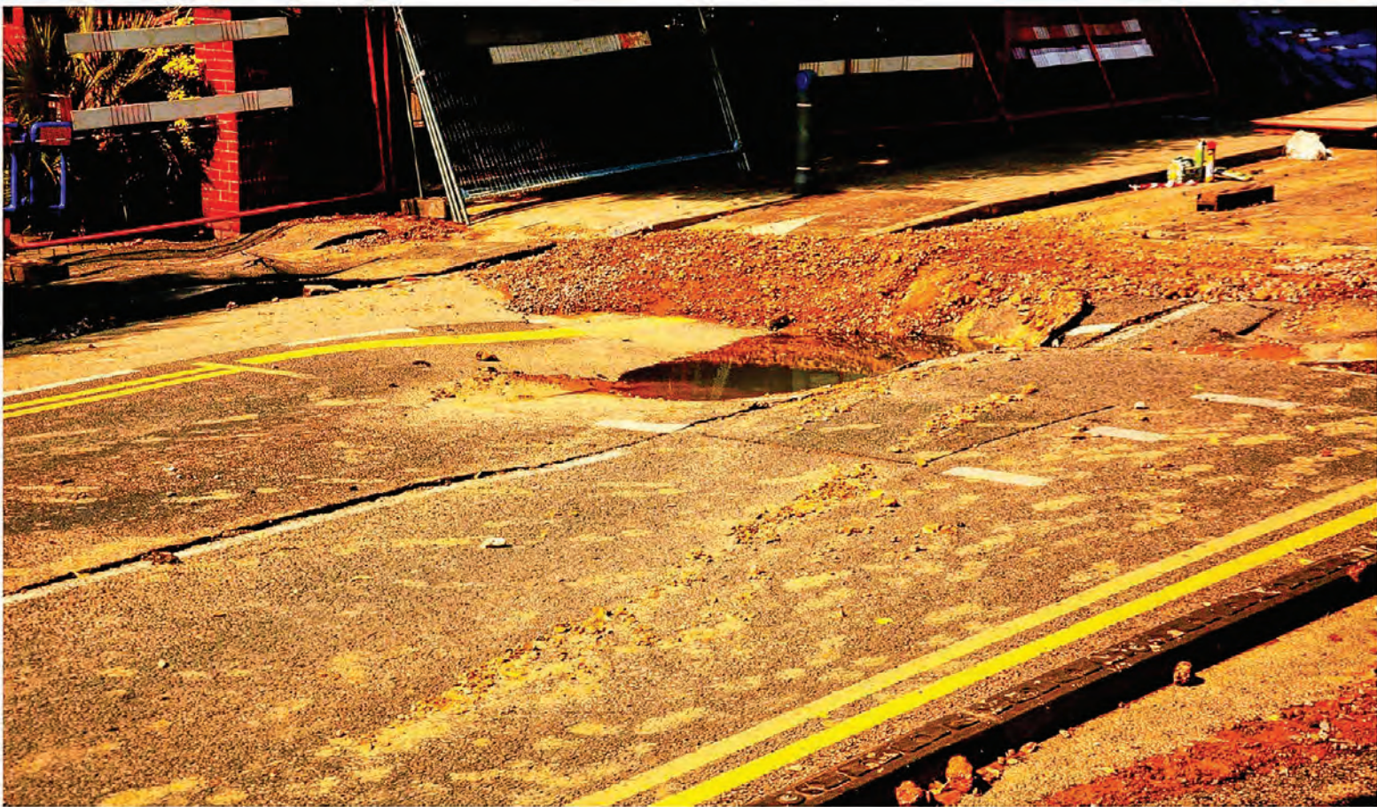
A heat wave in July 2022 caused major cracks in a roadway in Kingston upon Thames, a town in Greater London. Concrete expands in high heat, as do many other materials crucial to infrastructure and technology. Engineers and materials scientists are studying ways to manage increasing temperatures, including how to capture and reuse expended heat from machines and other devices.
