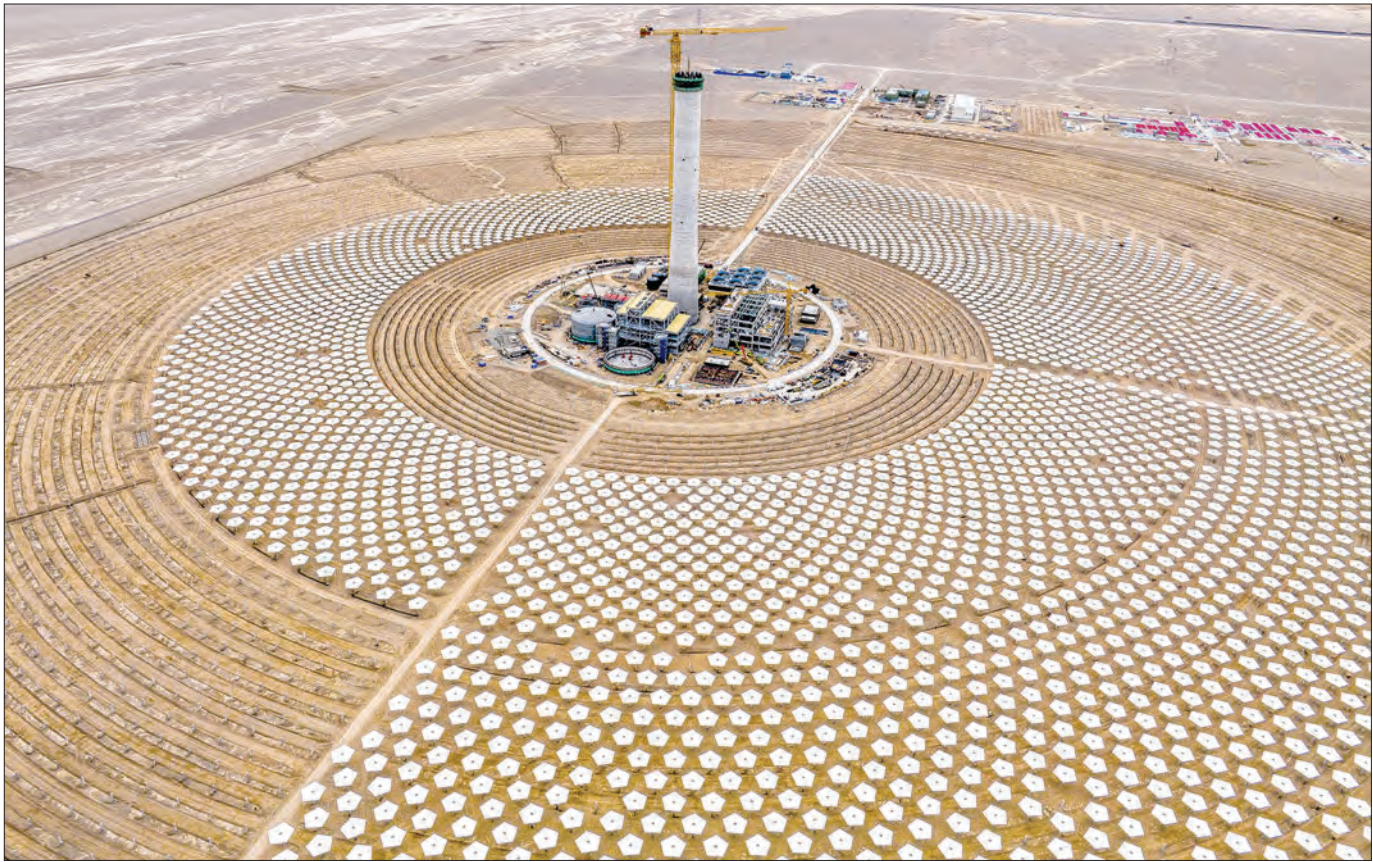
This aerial photo taken on 19 September 2023 shows a solar photovoltaic power project under construction in Zhangye, in China's northwestern Gansu province. PHOTO: AFP
