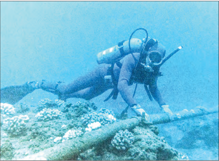
Diver checking underwater protection of cable. PHOTO: CC BY 2.0 / THE OFFICIAL CTBTO PHOTOSTREAM / SPUTNIK
