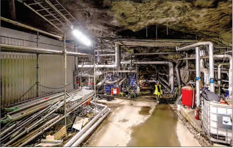
A worker walks at the site of a former oil storage cavern on 11 August 2023 in Västerås, Sweden, which is repurposed by Swedish energy company Mälarenergi and to be turned into a hot water storage facility. Mälarenergi, a Swedish energy company that provides various energy services to the region surrounding Lake Mälaren, is repurposing the former oil storage cavern into a massive energy storage facility for district heating, set to become Europe’s largest hot water storage at temperatures reaching 95 degrees Celsius, with a capacity of 300,000 cubic metres, upon its 2024 completion. PHOTO: AFP
