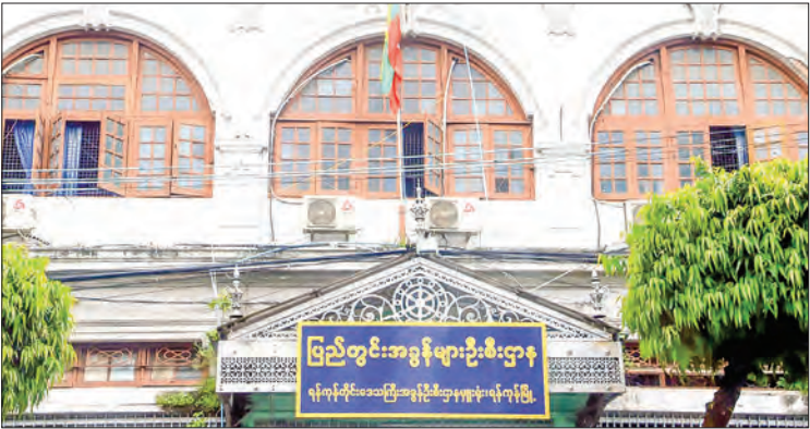
The general view of the IRD Office.
