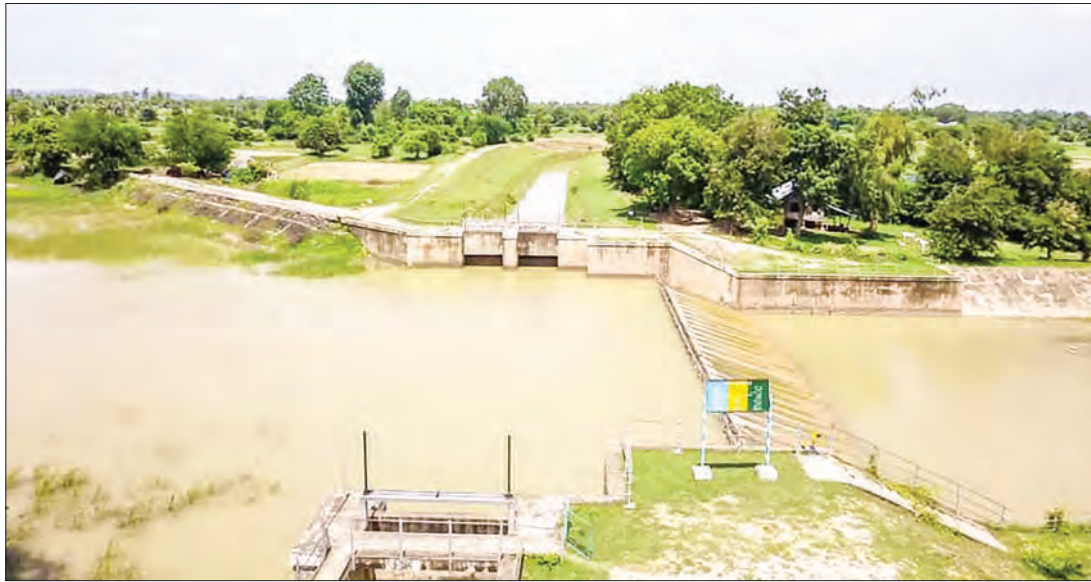
The view of Chaungmagyi Dam.
