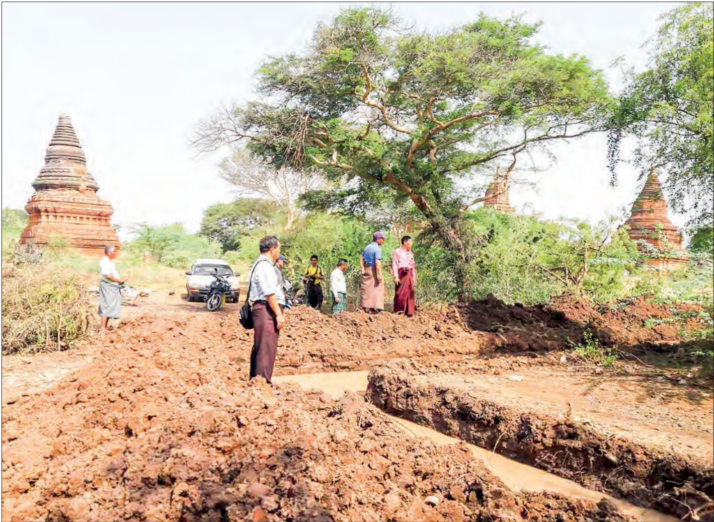
Maintenance of inlet and outlet drainage channels in the Bagan World Heritage Site in progress to solve the flooding in the region and future preventive measures.
