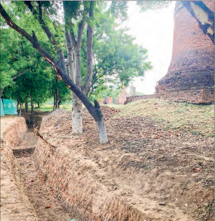
Maintenance of inlet and outlet drainage channels in the Bagan World Heritage Site in progress.
