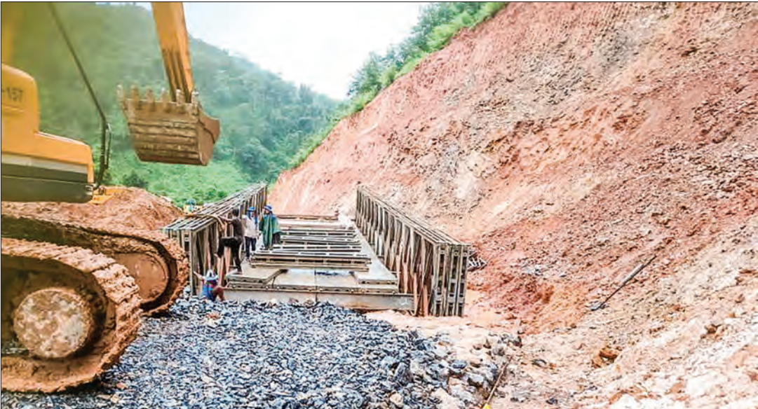
Progress underway: Construction of Bailey bridge in full swing.
