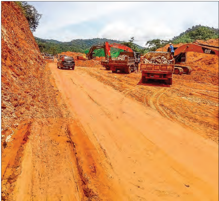
Road section undergoing repairs: Transformation in progress.
