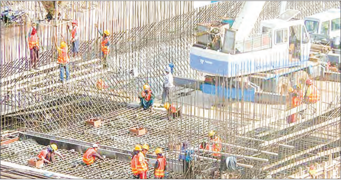
The concrete work for the outlet channel in the Shweli-3 Hydropower Project in Progress.
