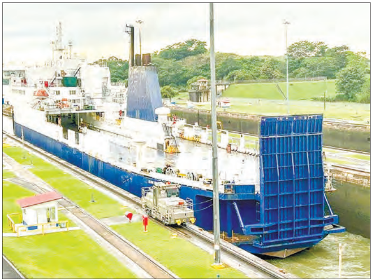
The canal relies on rainwater to move cargo ships through a series of locks that function like water elevators, raising the vessels up and over the continent between the Atlantic and Pacific Oceans. PHOTO: AUTONOMOUS EXECUTIVE PORT COMMISSION OF EL SALVADOR/AFP/FILE
