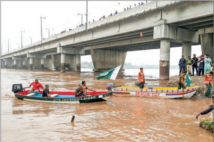
Pakistan’s civil defence rescue workers monitor the flood-affected river Ravi in Lahore on 16 July 2023. PHOTO: AFP
