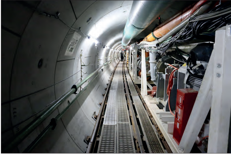
Photo shows an undersea tunnel to be used to discharge treated water from the crippled Fukushima Daiichi nuclear power station in Japan's northeast. PHOTO: TOKYO ELECTRIC POWER COMPANY HOLDINGS INC. /KYODO
