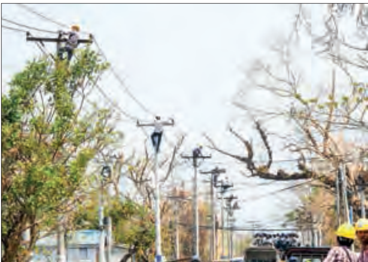
MoEP staff are seen repairing cables yesterday.
