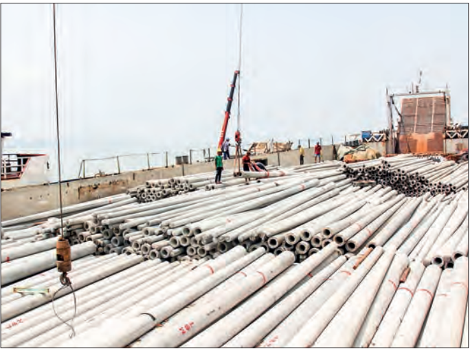
Unloading of concrete lamp-posts
