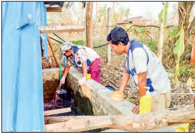
Water chlorination in Ponnagyun Township.
