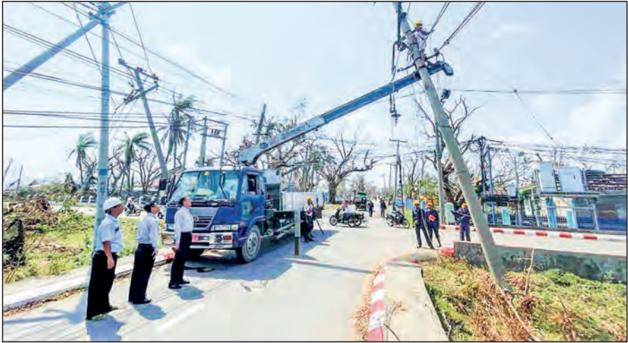
The re-erection and reinstallation of electricity poles and power cables underway in Sittway.
