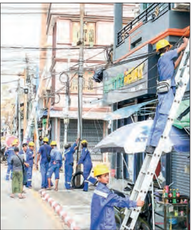
Communication cables are re-installed.
