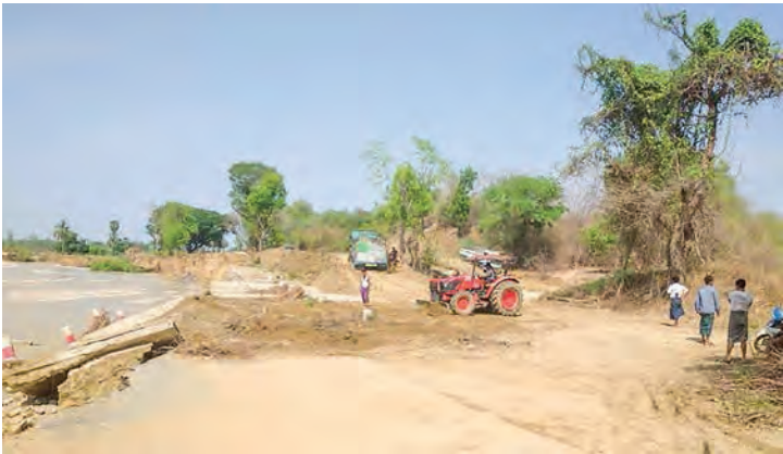
Roads eroded by Chitchaung in Seikpyu Township.
