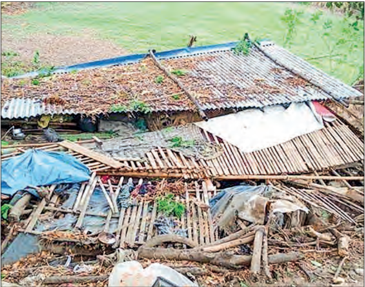
Debris in the aftermath of Cyclone Mocha.
