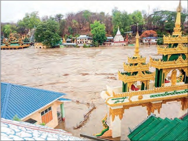
Flash floods in Mann Shwesettaw Pagoda.
