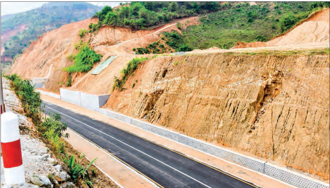
The construction site of the Kengtung detour.
