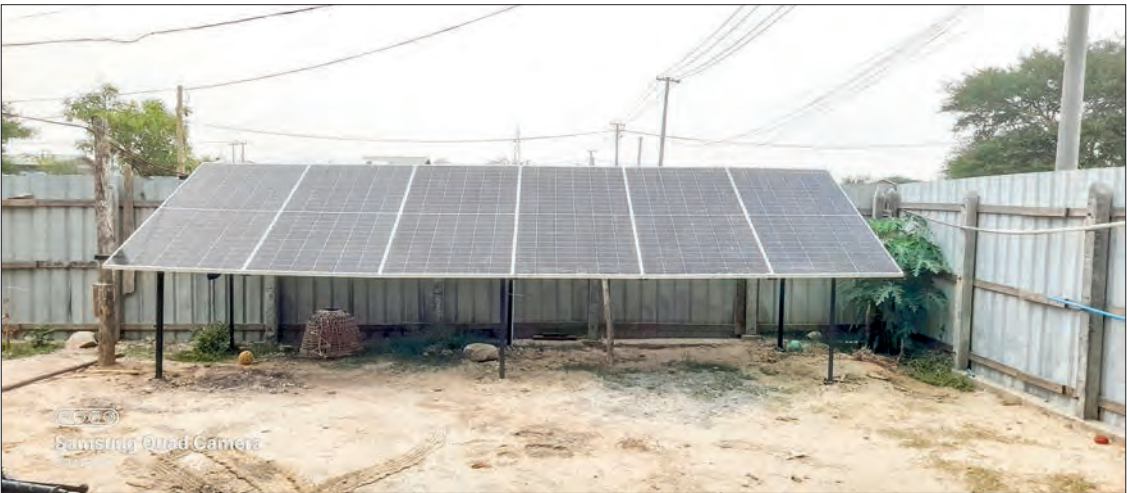
A solar panels installation.
