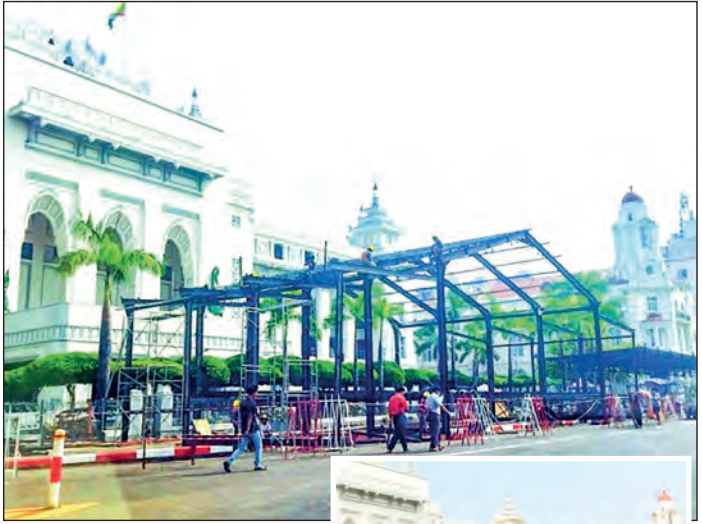
Yangon Mayor's Maha Thingyan Water Festival pandal under construction.
