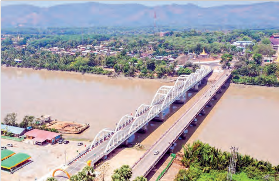
An aerial view of already-opened Kamyawkin Bridge.
