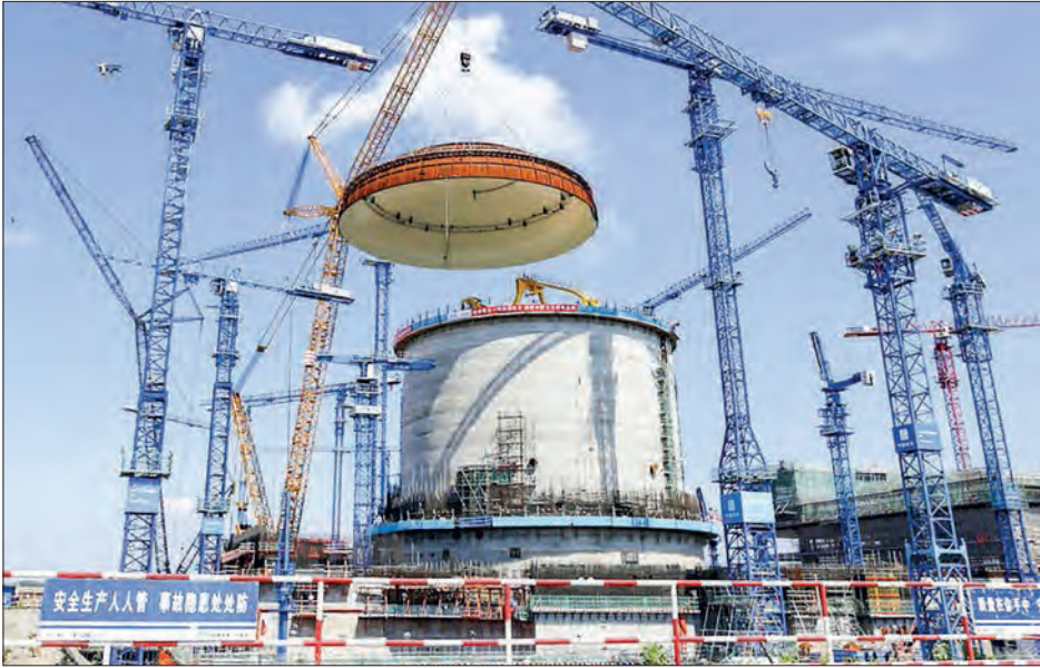
Photo taken on 23 May 2018 shows the installation site of a hemispherical dome at the No. 3 unit of Fangchenggang nuclear power station in south China's Guangxi Zhuang Autonomous Region. PHOTO: FANGCHENGANG NUCLEAR POWER CO., LTD/XINHUA
