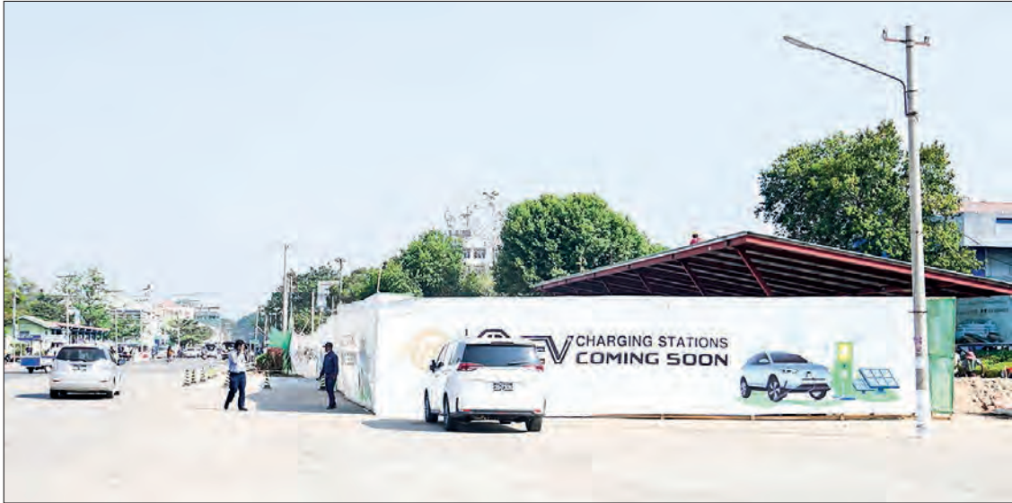
EV charging stations are under construction.
