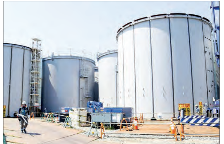
Photo taken 26 August 2020, at the crippled Fukushima Daiichi nuclear power plant in northeastern Japan, shows tanks for storing treated water from which most of the radioactive contamination has been removed.
