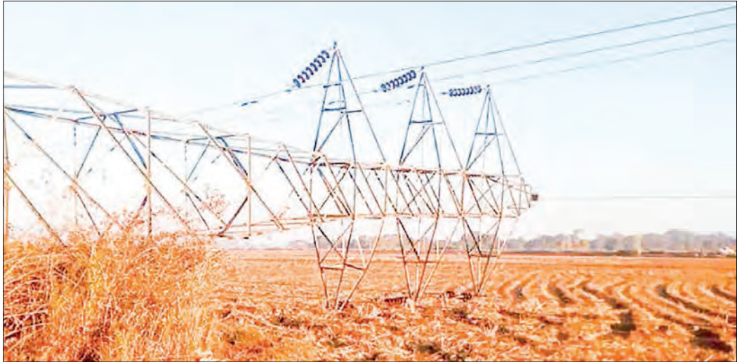
A photo shows fall of tower for 132KV Biluchaung(2)-Tikyit double power cables.
