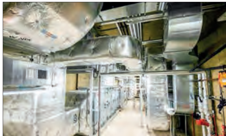
This energy-efficient system sucks warm air from outside to heat air/water inside the building. PHOTO: AFP
