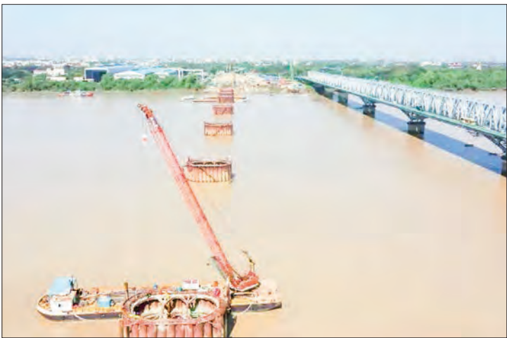
A new Thanlyin Bridge is under construction.
