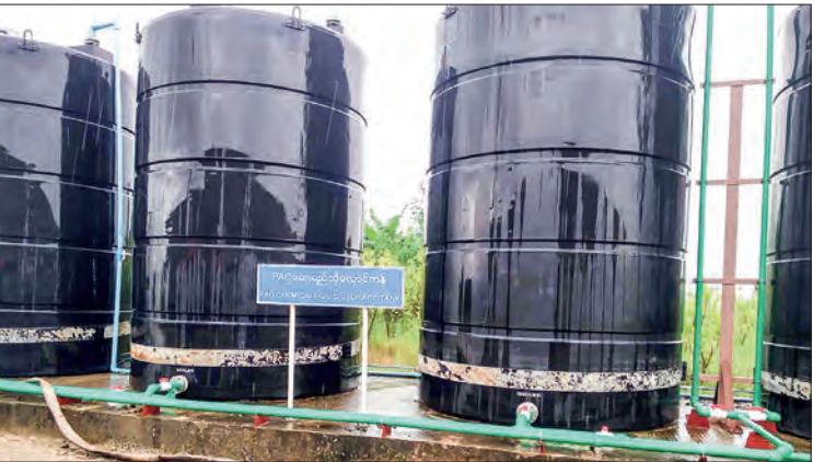
PAC Chemical Liquid Storage Tank at Ngamoeyek Water Treatment Plant (Nyaungnapin).
