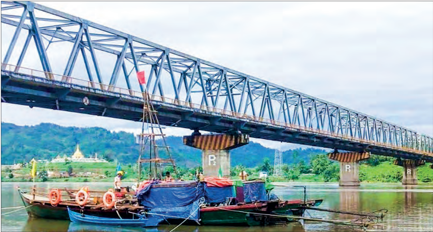
The new No 2 Bala Minhtin bridge is under construction across the Ayeyawady River.
