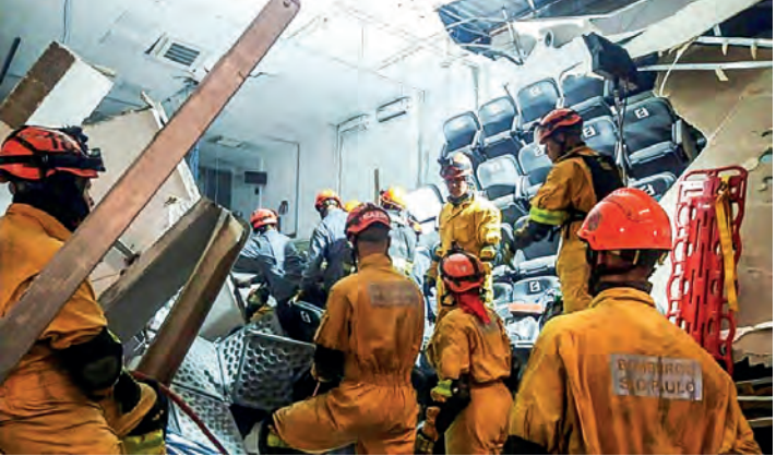
Handout picture provided by the official Twitter account of Sao Paulo fire department showing firefighters working inside a collapsed building in Itapecerica da Serra, Sao Paulo state, Brazil, on 20 September 2022. PHOTO: AO PAULO FIRE DEPARTMENT/AFP
