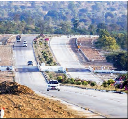
One section of the Yangon-Mandalay Expressway.
