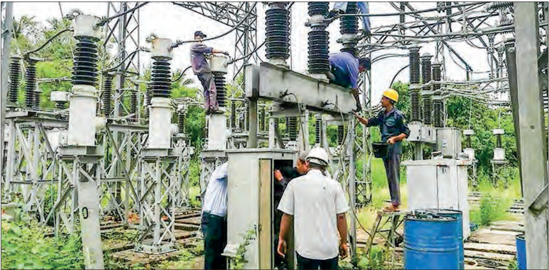
Workers repair electric transformers. PHOTO: YESC
